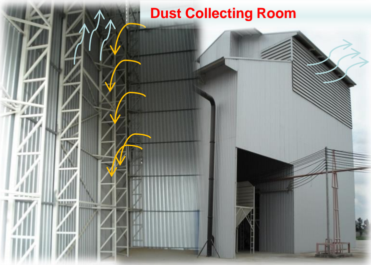
Clean Air exhaust to atmosphere
